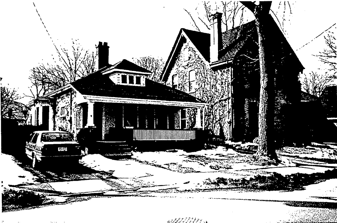
Photographs 5 (top) and 6 (bottom) show the major differences between the two eras of original construction and later remodelling in 7 and 9 Prospect.
