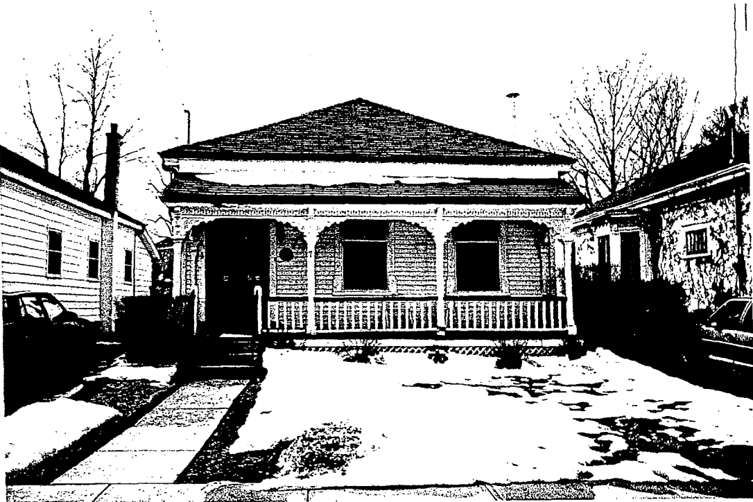
Photographs 1 (top) and 2 (bottom) show the facades of 5 and 7 Prospect respectively. Note the difference in verandah, balustrading and windows.
