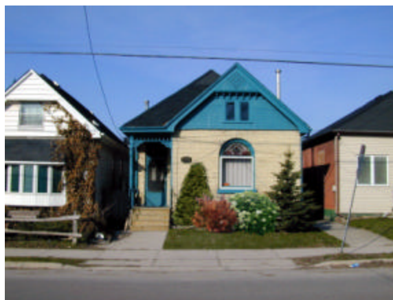
Front yard available for landscaping if parking on street was permitted
