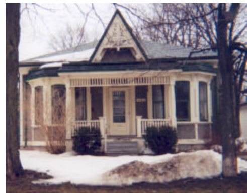
Distinctive front porch with decorative spindles and columns
