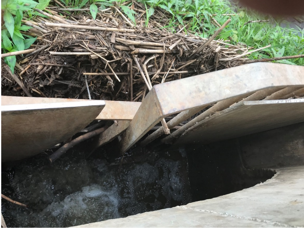
Powell Drain Culvert Orifice – Weir Structure
