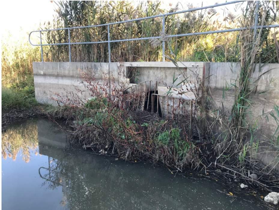
Powell Drain Culvert Orifice – Weir Structure
