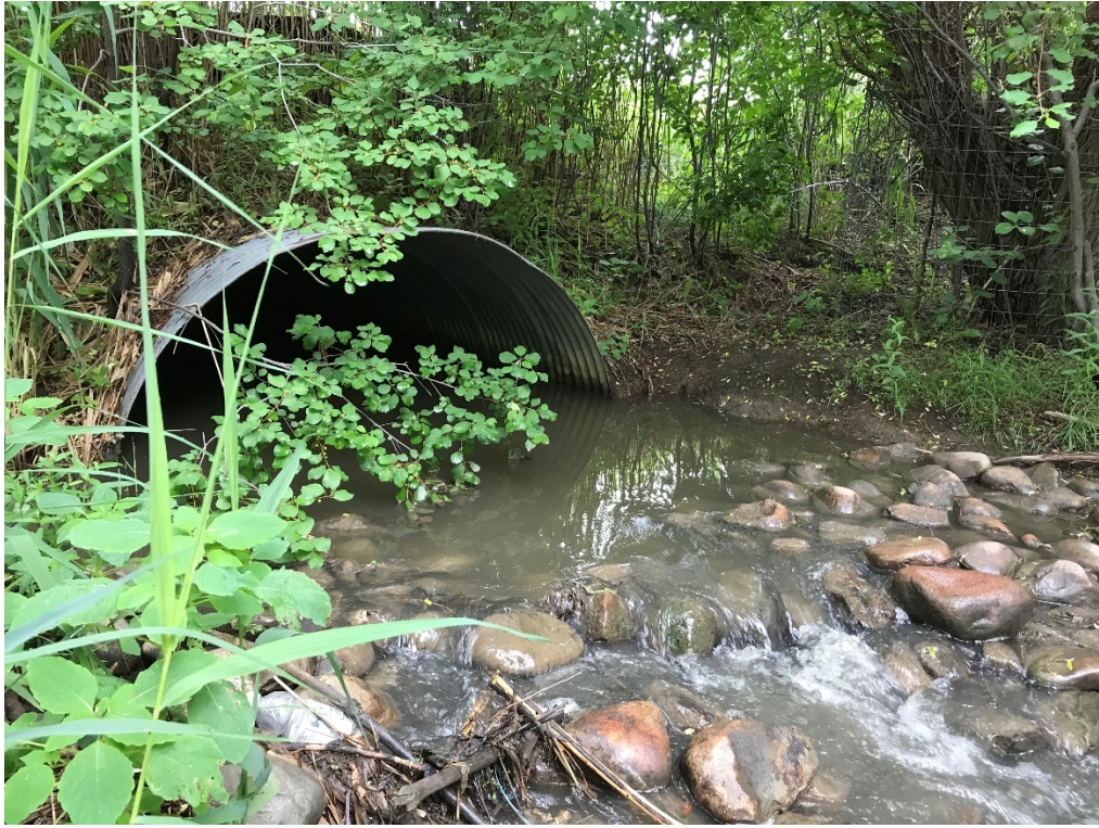
Powell Drain Culvert Outlet
