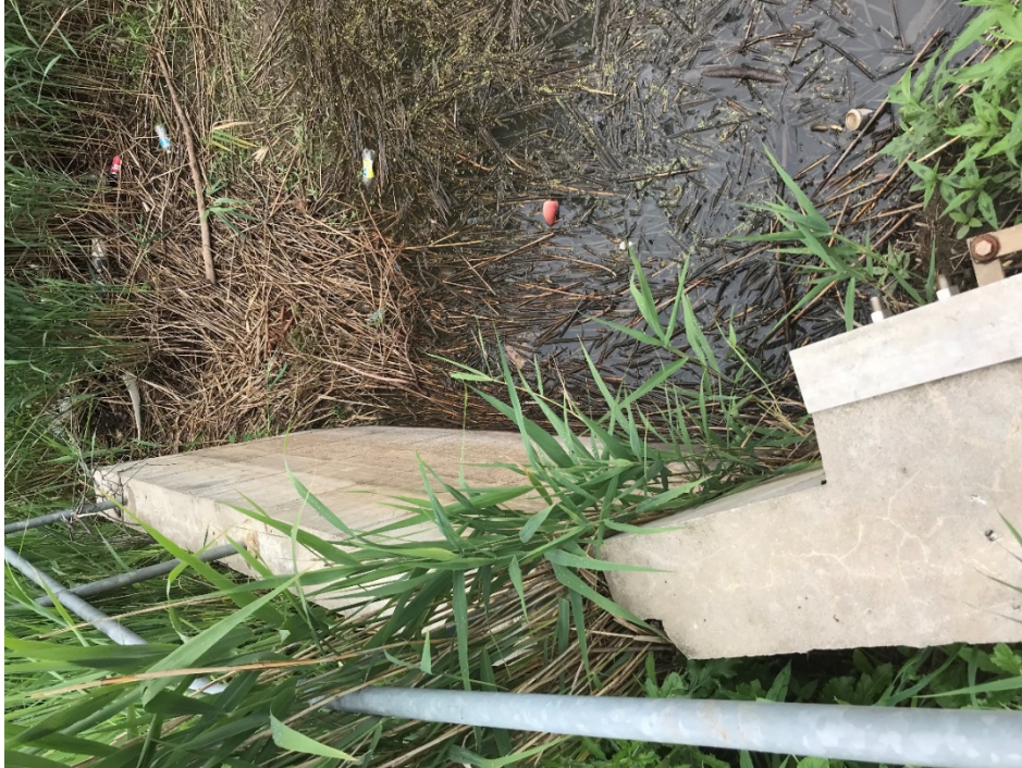
Powell Drain Culvert Headwall
