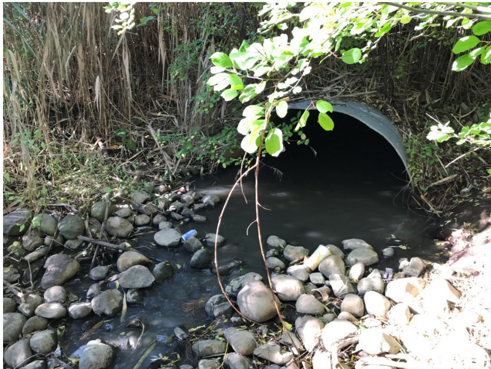
Powell Drain Culvert Outlet
