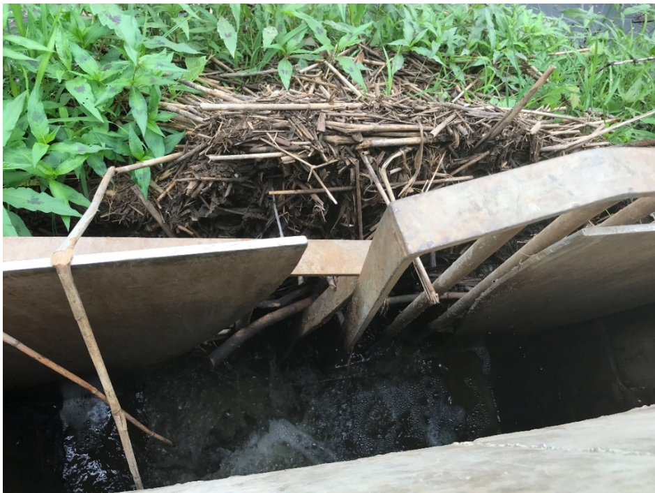
Powell Drain Culvert Orifice – Weir Structure
